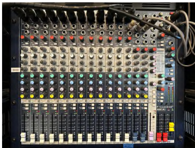
Sound System in Meeting Room K
